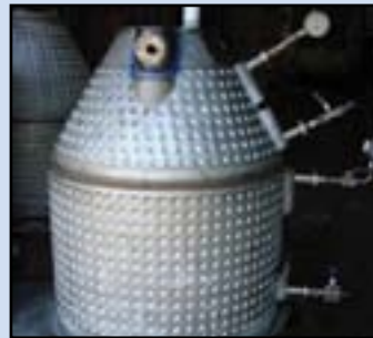
Pressure testing dimple jacket of contramix vessel
