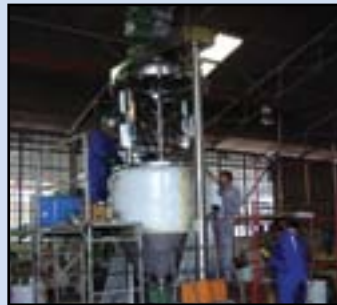
1250 ℓ Contramix vessel raise/lower being tested
